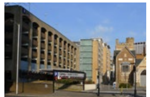
Existing car park and vehicular entrance
