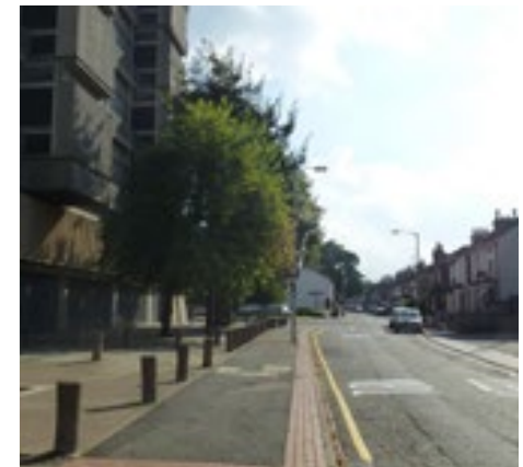
The existing public realm is of mixed quality along Church Road
