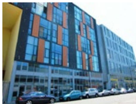
Issigonis and Morris House, Acton - live/work units which provide activity to the street
