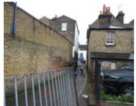
The existing Drummond Road Car Park and the pedestrian route to Church Street
