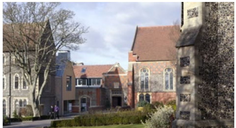
Woolton Quad, Brighton College; sensitive new building in a historic context
