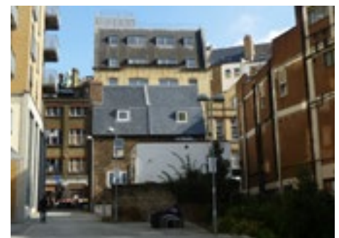
View in the square looking east - existing public realm at Exchange Square includes some planting in the form of a green wall which creates a barrier in the square. There is a change in level, rising towards Surrey Street
