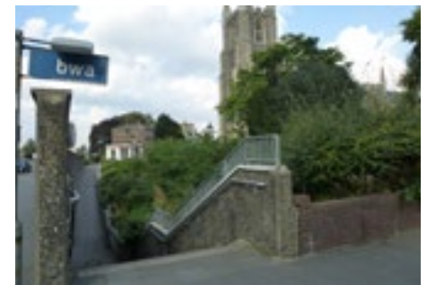
The existing subway does not create a pedestrian friendly public realm along Roman Way
