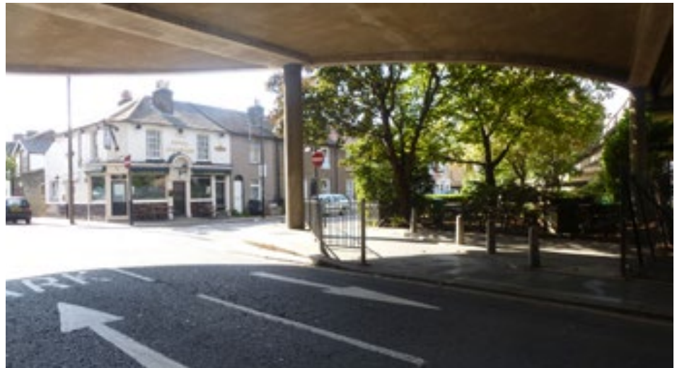
Existing Croydon Flyover undercroft with the beer garden of the Royal Standard
