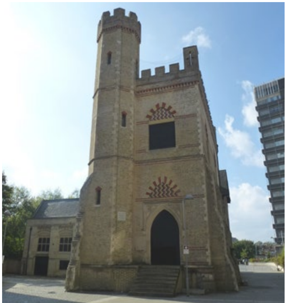
Surrey Street Pumping Station, Exchange Square
