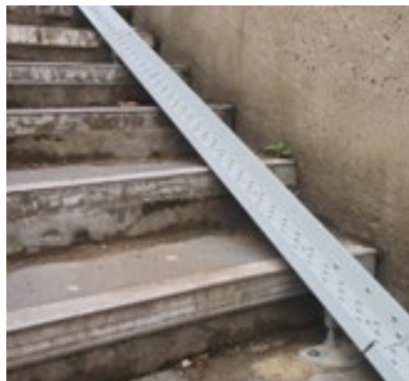
Wheeling channels, Old Barn Lane, Croydon
