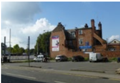
The existing Ann's Place car park and Eagle Pub
