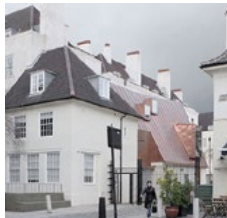
New Horizon Youth Centre, Somers Town, North London with copper extension (Adam Khan Architects)
