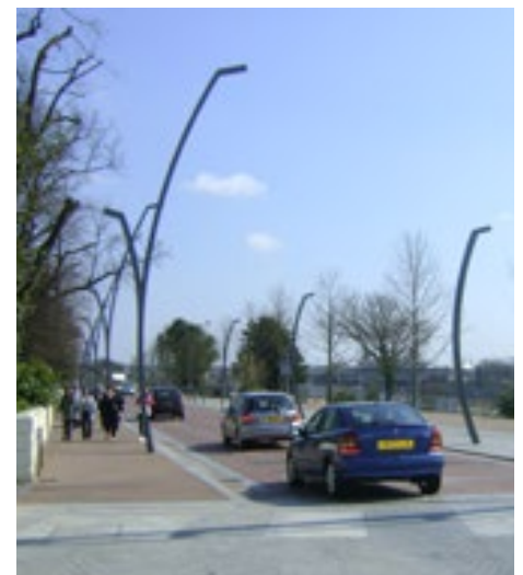
Shared surface treatment of the town’s southern ring road. Space has been given back to pedestrians and used to plant street trees, Ashford.
