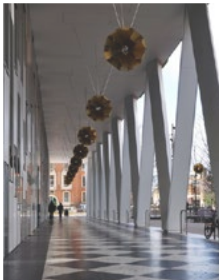
Attractive and creative lighting and paving at Barking Town Square
