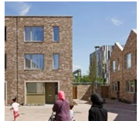
Ann Mews, (MaccreanorLavington). Attractive family homes with doors to the street
