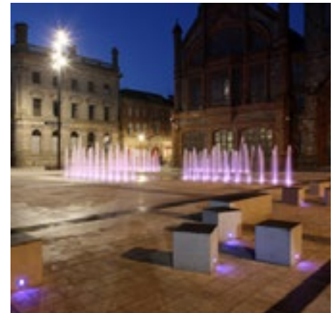
Public realm sympathetic to its historic context with new seating and lighting. Derry Guildhall Square (BDP).
