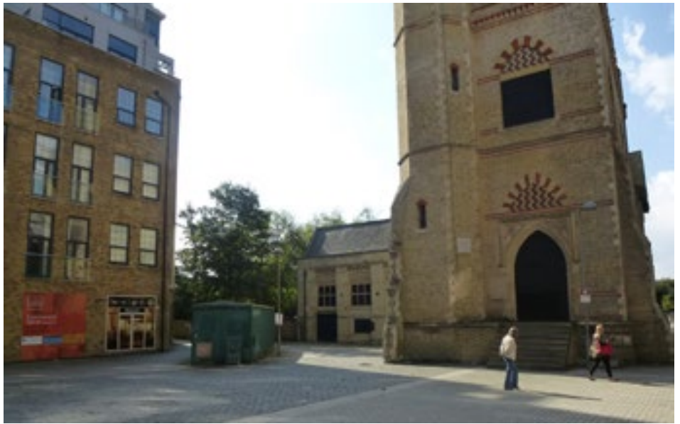
Surrey Street Pumping Station in Exchange Square
