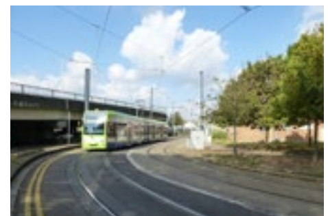
Existing tramways and the jubilee flyover
