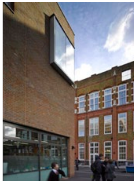
A new extension and new buildings at a Victorian School building for the Aylesbury Academy, London
