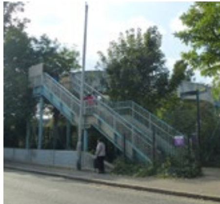
The existing bridge into Wandle Park
