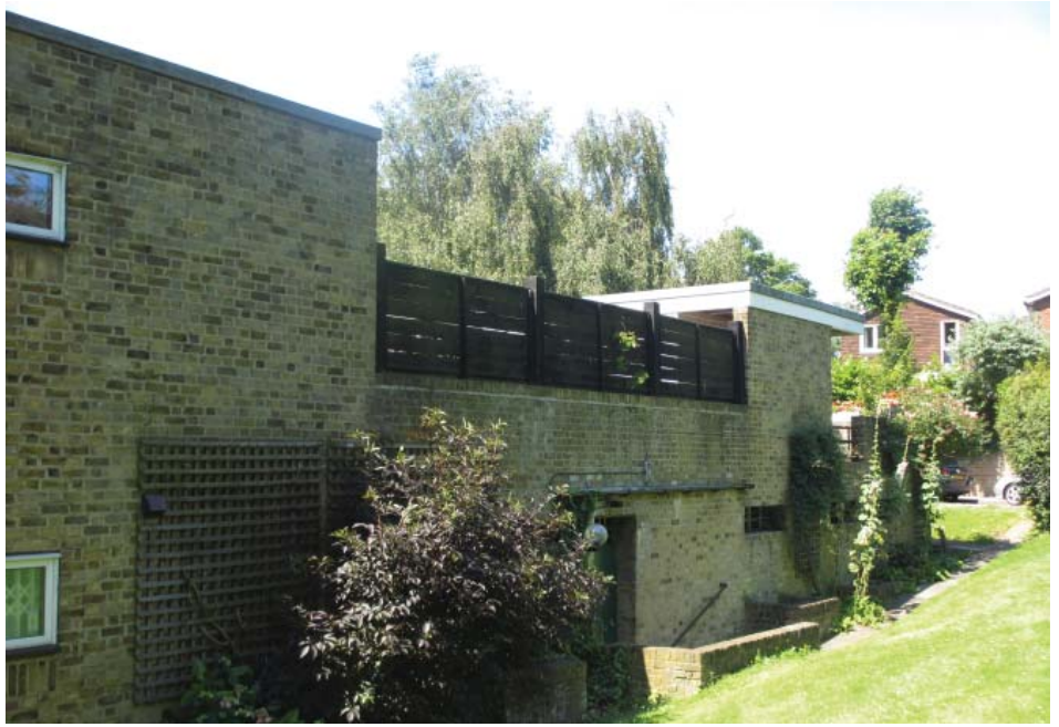
The north-east elevation of a terrace, showing the porch structure to the right and fenced upper garden between that and the main house
