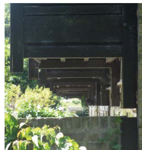
The underside of balconies
