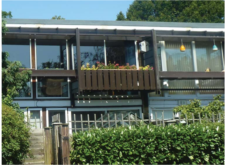
Timber balconies along a terrace at St Bernards
