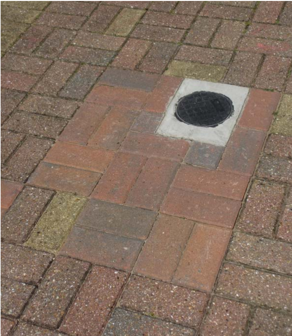
Examples of mismatching materials that have been replaced following works carried out by third parties
