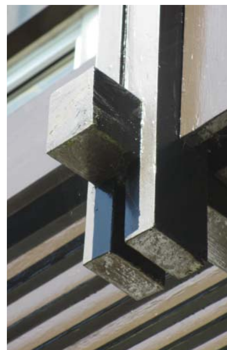
An example of the high quality construction detailing present
