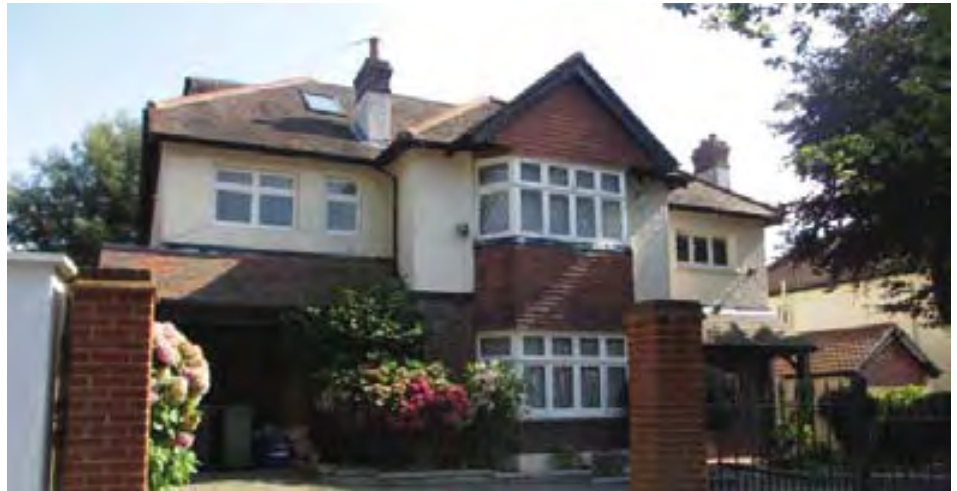
Two storey extension to 60 Ryecroft Road, set back from the front wall
