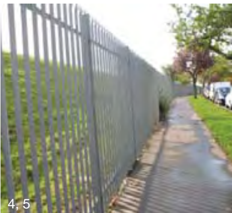
Palisade fencing on Ryecroft Road
