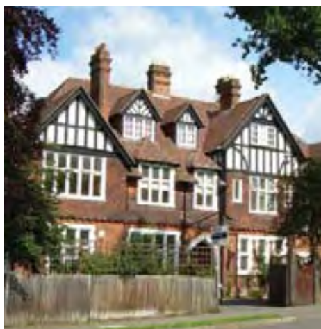
Number 69 Ryecroft Road, larger in scale and bulk than most other buildings on the road
