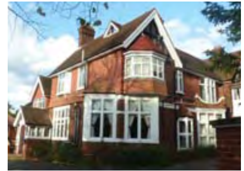
Gibson's Lodge Nursing Home - the building has been substantially extended to the south-west
