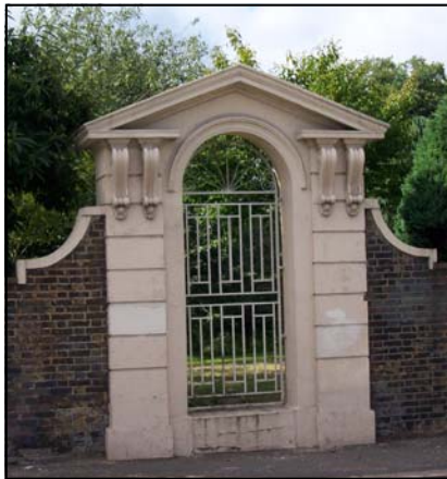
Westow Park Arch, Church Road, South Norwood
