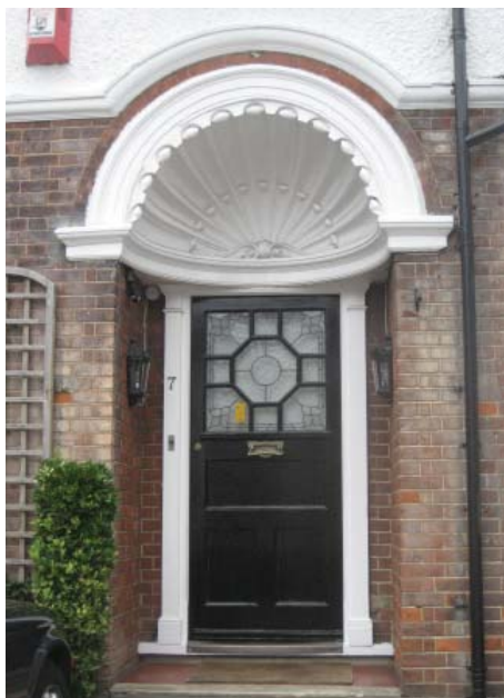
Shell niche doorway at 7 Eden Road
