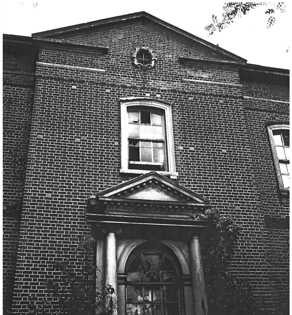
Historic photograph of Grove House c.1952-3
