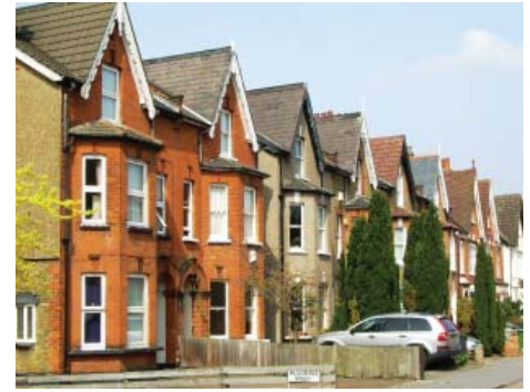
An example of the consistent pattern of rooflines present in the area
