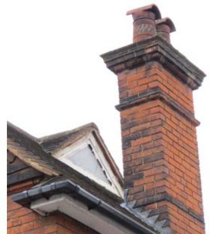
Chimney and gablet at 53 Chatsworth Road
