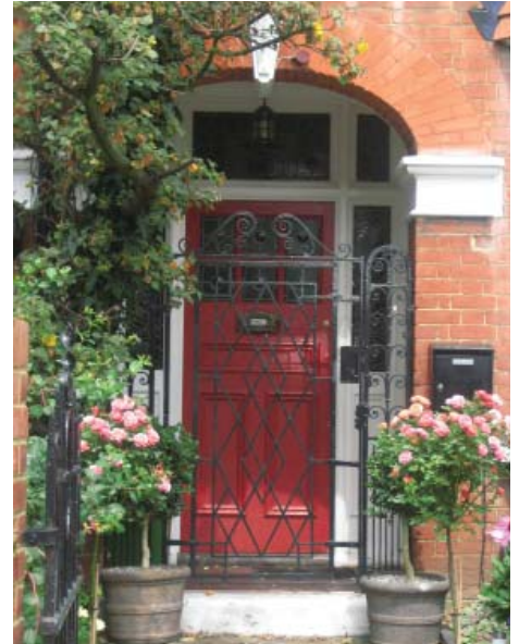
Recessed porch with iron gate for extra security, an acceptable alternative to the solid infilling of the porch
