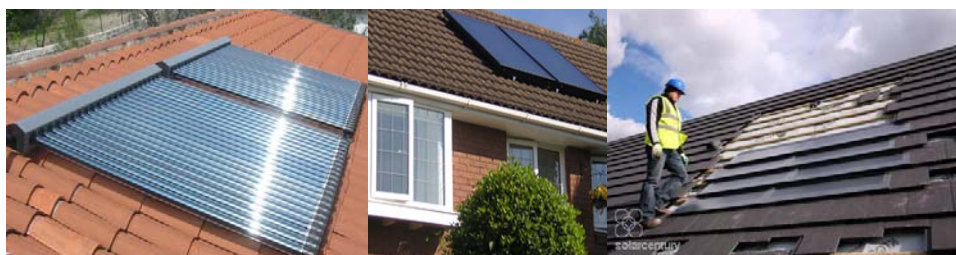
Figure 29: Solar collectors (l-r): Evacuated tube, flat plate and tile (Sources: Riomay, generateyourown.co.uk, Solarcentury)
