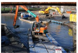
The Environment Agency funded a dredging programme which was completed in early 2009. The task to remove urban sediment and other matter from the canal over a distance of 3.2kms was completed over a 3 month period at a cost of £2million. As a result of the initiative over 30,000 m3 of sediment was removed in addition to 3 tonnes of tyres, 3 cars, 40 motorbikes and 120 shopping trolleys.
