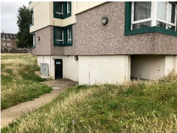
Fig 7 Low level south-eastern elevation 2-56A Showing render finish to ground floor to concrete and brick substructure
