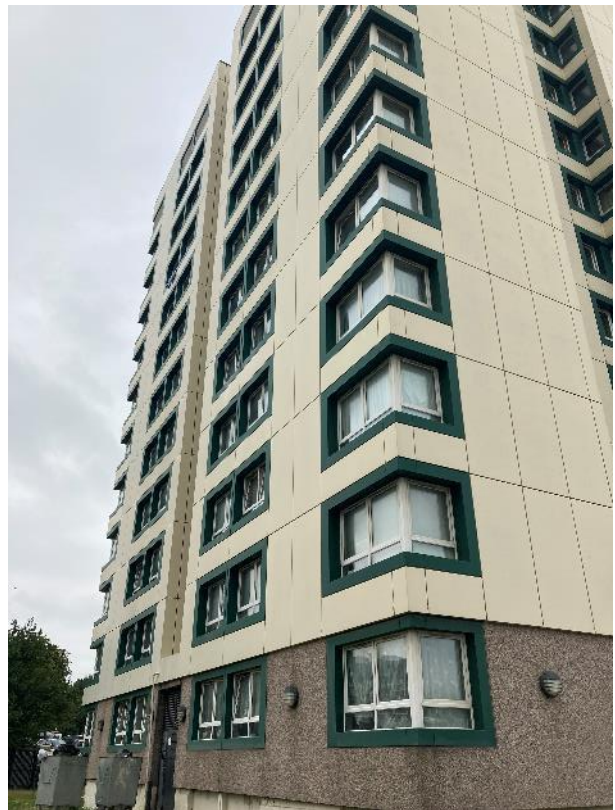
Fig 6 View of Northern elevation 2-56A
