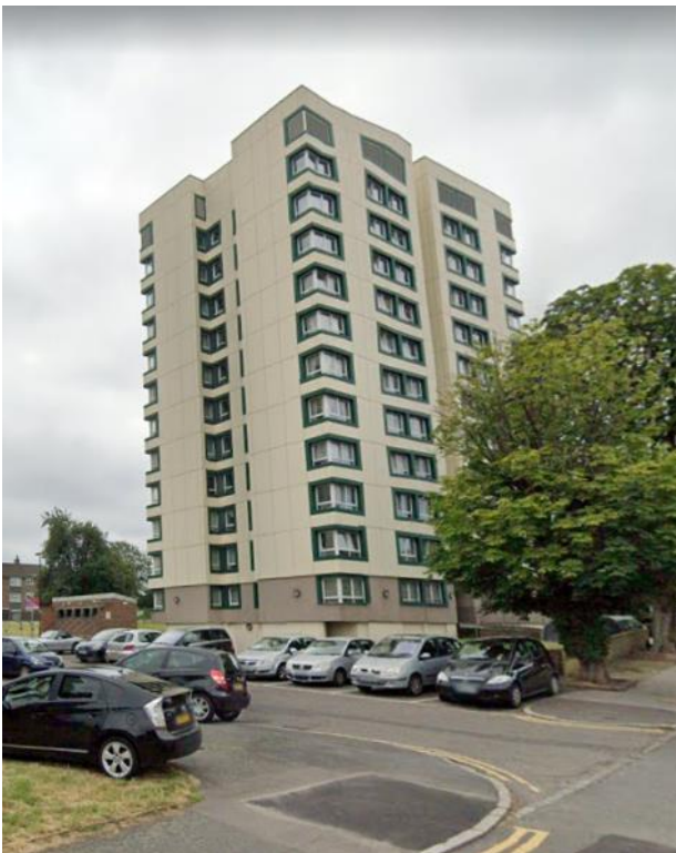
Fig 1 View of South and West elevations of 2-56A
