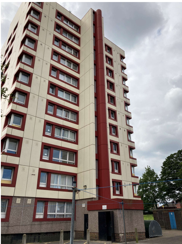
Fig 2 View of Northeast elevation showing waste chute Added after original construction
