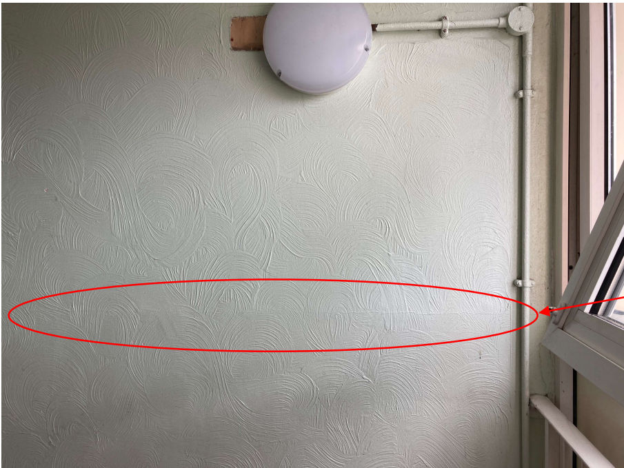
Fig 6 Horizontal joint between wall units just visible in plaster
