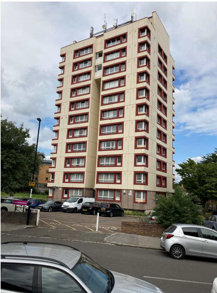
Fig 1 View of Southeast elevation of 1 to 87 Regina Road
