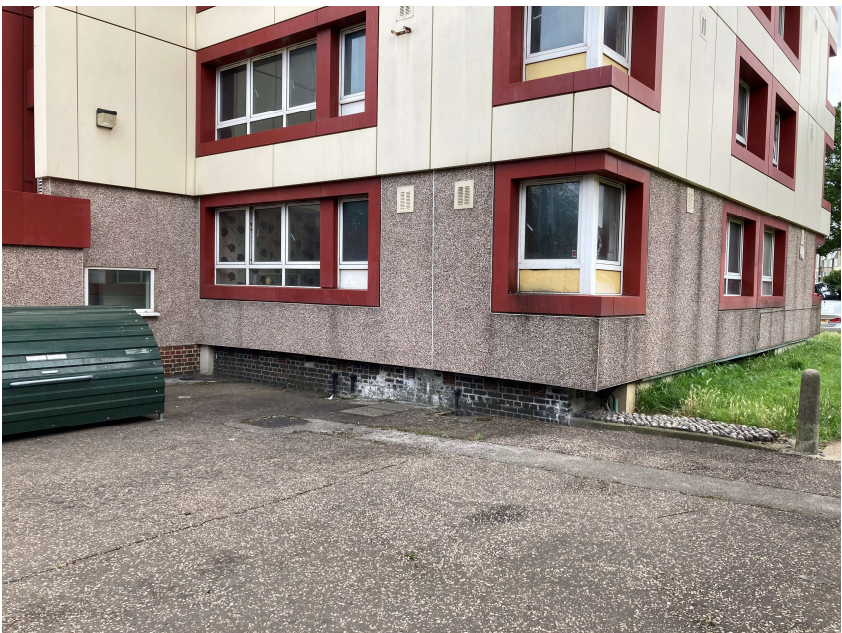
Fig 3 Showing render finish to ground floor to over-cladding and aluminium panels used for remainder of block
