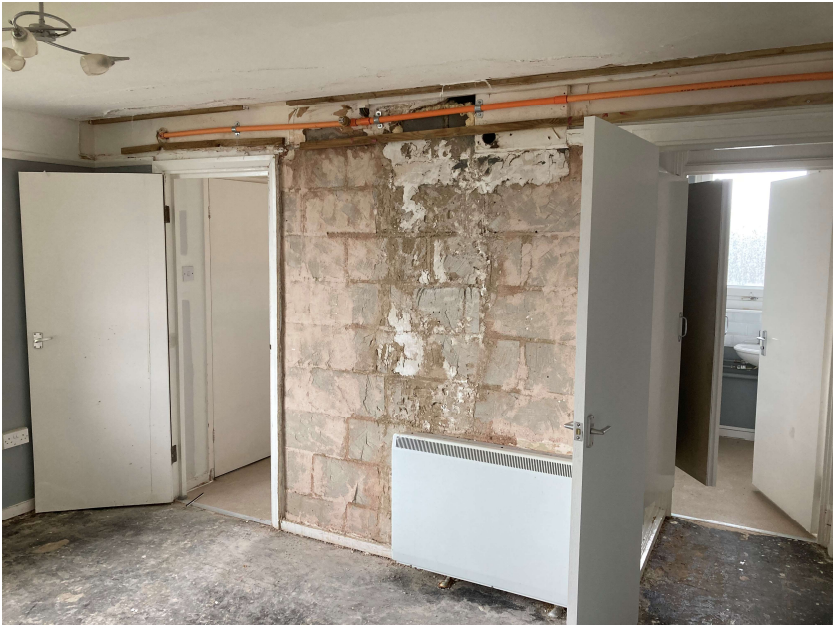
Fig 5 Showing blockwork partition within flat
