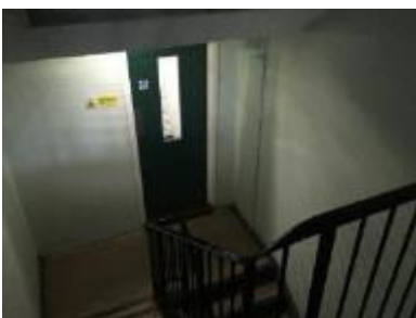
Figure 23 Stairwell with general lighting on.
