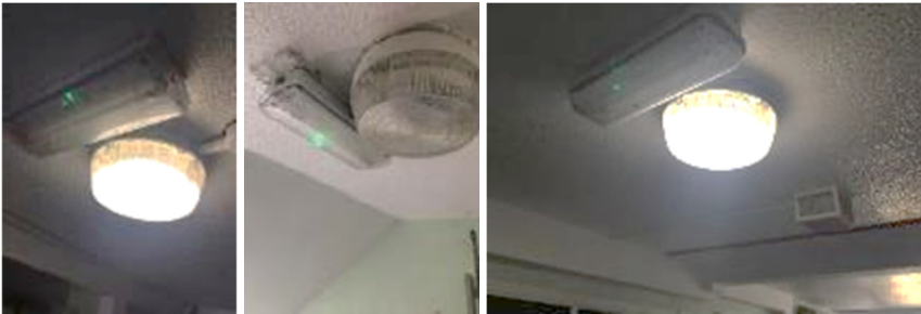
Figure 22 Ground floor rear corridor.
