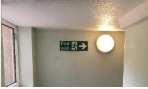
Figure 21 Ground floor rear corridor.
