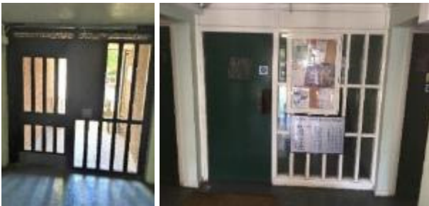
Figure 25 No directional signage from lift lobbies.
